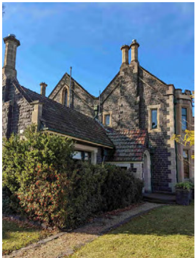
Figure 6 View of gatehouse from south-west showing small gate and pathway
