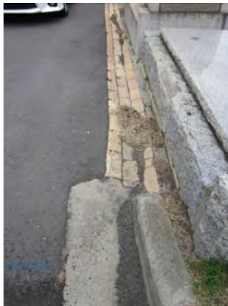
Figure 4 Apricot three brick channel to the west side of South Avenue Source: 2014 CMP
