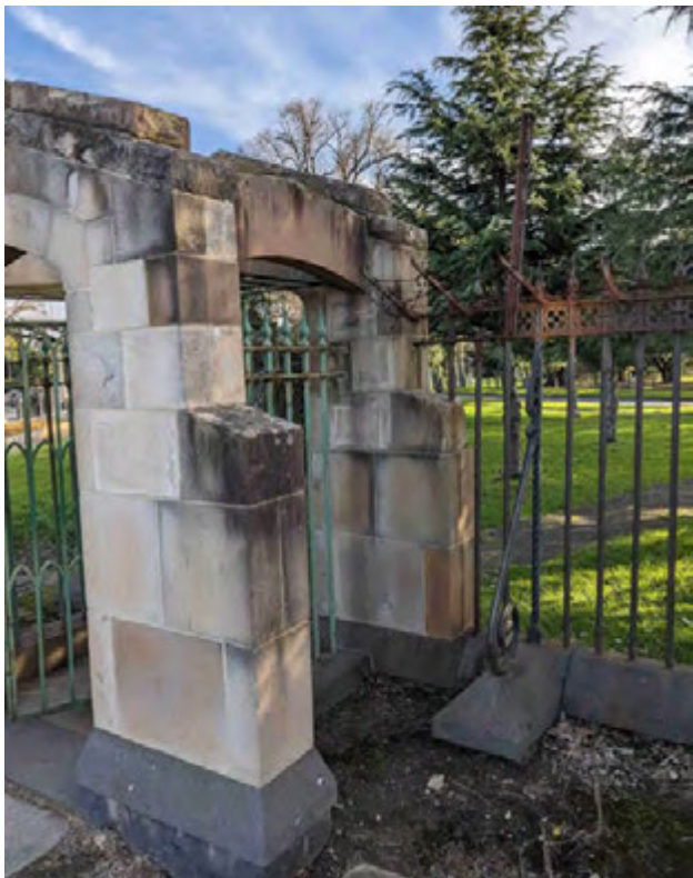
Figure 3 Northern view of gate and enclosure
