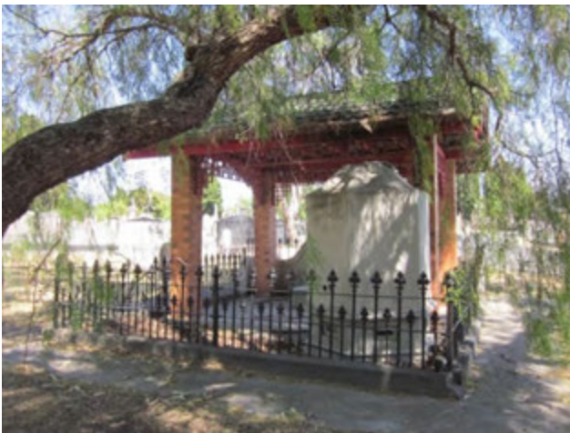
Figure 3 West view of the enclosure showing the rear of the funerary oven Source: 2014 CMP
