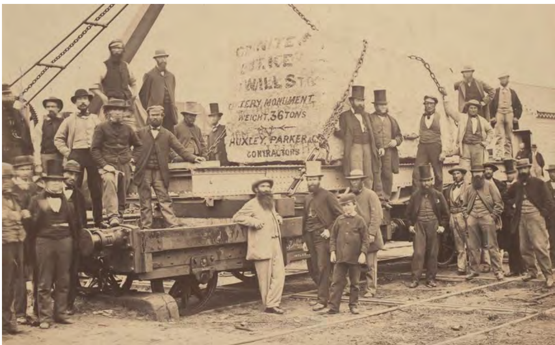
Figure 36 Delivery of the block of granite for the Burke and Wills memorial, 1864 Source: Charles Nettleton collection, State Library of Victoria
