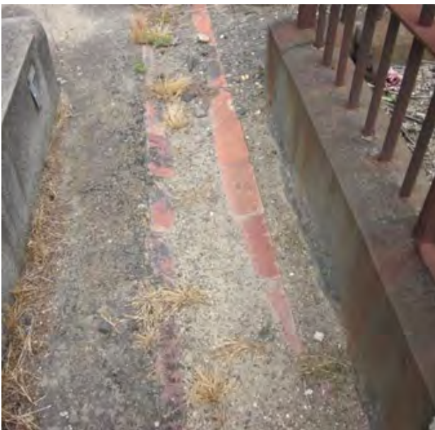
Figure 3 Remnant section of three brick channel between graves Source: 2014 CMP
