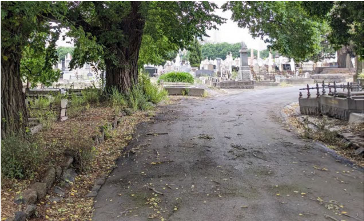
Figure 1 Roadway retaining original bluestone channels
