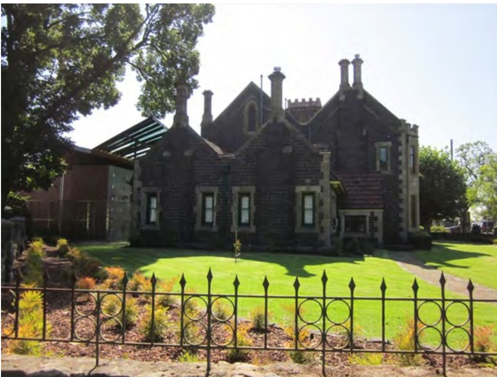
Figure 2 Gatehouse viewed from the west with wrought balustrade in the foreground
