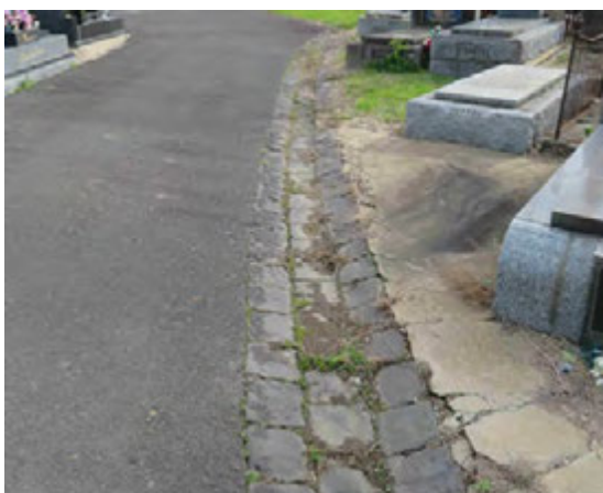
Figure 50 Drainage: (upper left) remnant three brick channel between graves (2014); (upper right) junction of concrete drains; (lower left) remnant three-pitcher bluestone channel; (lower right) remnant four-pitcher bluestone channel, with new graves infilling the roadway
