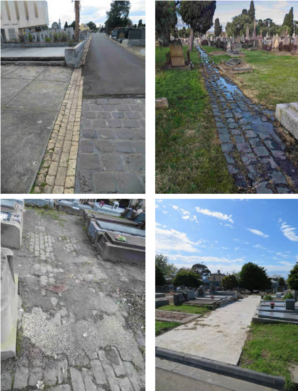
Figure 51 Paths and interfaces: (upper left) bluestone driveway from south-east gate leading to asphalt roadway, with brick channels; (upper right) bluestone pincer path; (lower left) remnant bluestone pincer path with deteriorating asphalt overlay; (lower right) new concrete path
