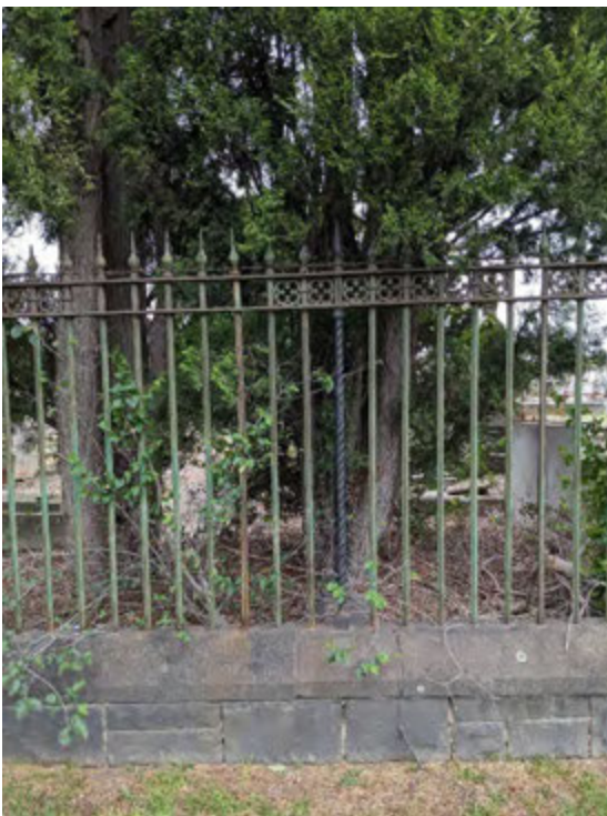
Figure 13 Infrastructure: (left) Cast iron palisade perimeter fence on bluestone plinth; (right) Early Drinking Trough at original (west) main entrance (now adjoining Melbourne Mausoleum)
