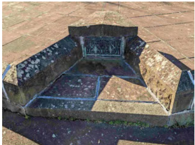
Figure 4 Low bluestone perimeter wall to the flagstone courtyard and raised ventilation shaft with decorative wrought grate to the crypts
