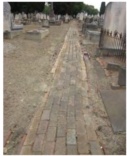
Figure 3 Brick path with terracotta channel west of Sixth Avenue looking west (CMP 2014)
