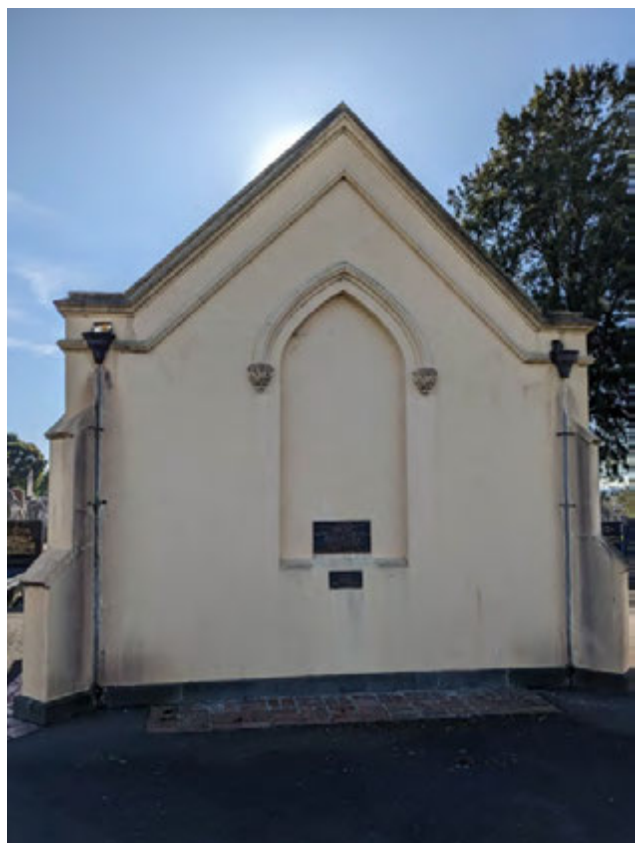
Figure 4 South elevation of Jewish Mortuary Chapel
