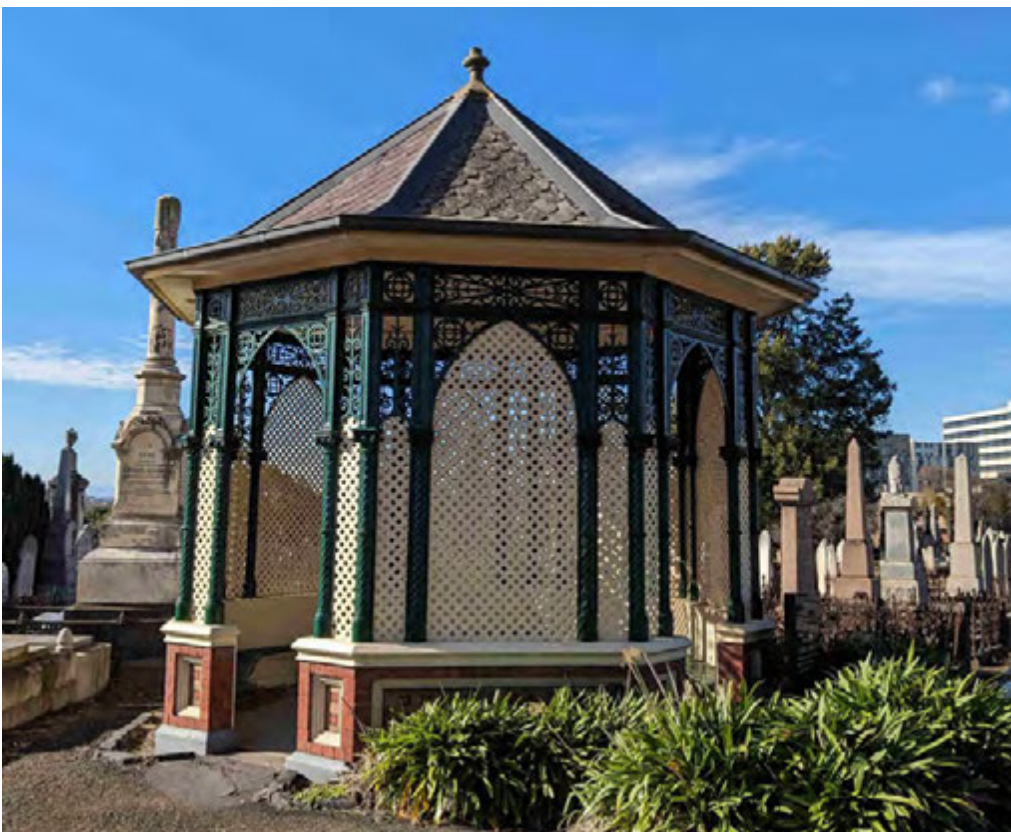
Figure 2 Rotunda no.2 on South and Second Avenues
