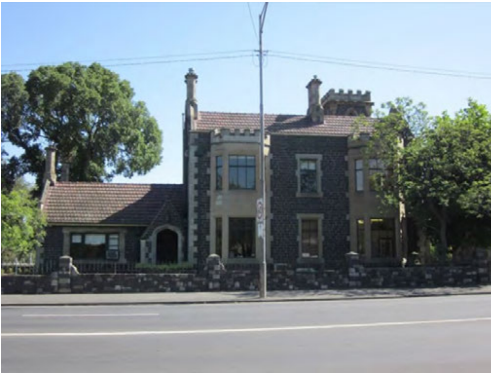
Figure 1 Gatehouse viewed from south side of College Crescent, set behind the random rubble stone wall
