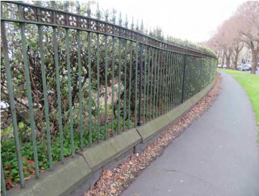
Figure 1 Perimeter fence with hedge as viewed to the south along Cemetery Road East
