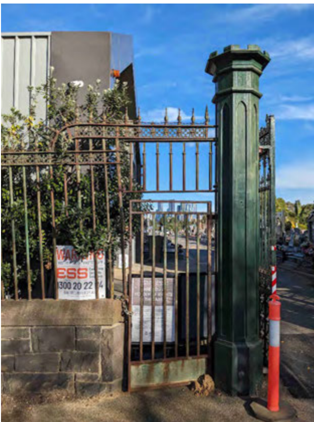
Figure 2 Eastern pedestrian gate
