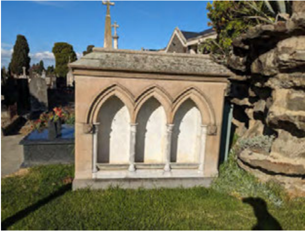
Figure 1 Front view of drinking trough showing stepped sloping roof, triple arched opening and marble insert for fonts and bluestone plinth (facing west)
