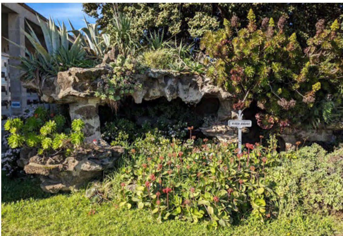
Figure 62 Remains of the southern large rockery today, showing the extensive loss of sections of the original structure, its fine geological details, and most of the lower water basins, coping and niches
