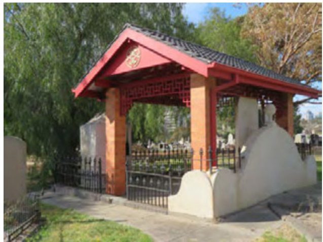
Figure 4 Modern shelter structure with rendered wall to east of enclosure
