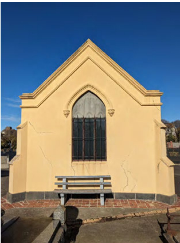
Figure 3 North elevation of Mortuary chapel
