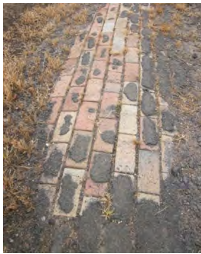
Figure 2 Brick path remnant with deteriorating asphalt overlay west of Second Avenue (2014 CMP)
