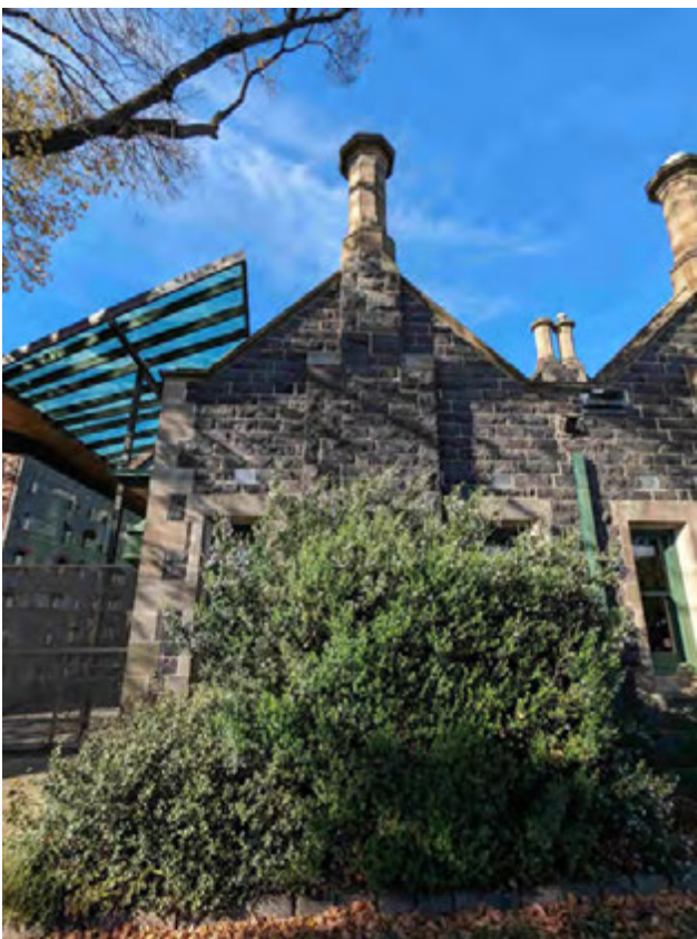
Figure 5 View of gatehouse from west with adjoining columbarium walls to the left
