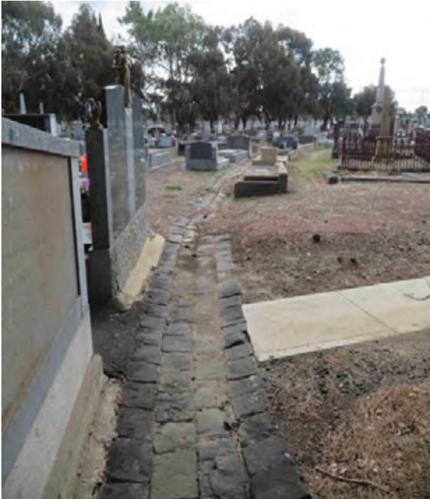
Figure 1 Remnant four-pitcher bluestone drainage channel
