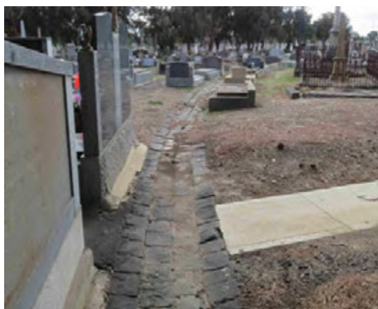
Figure 50 Drainage: (upper left) remnant three brick channel between graves (2014); (upper right) junction of concrete drains; (lower left) remnant three-pitcher bluestone channel; (lower right) remnant four-pitcher bluestone channel, with new graves infilling the roadway
