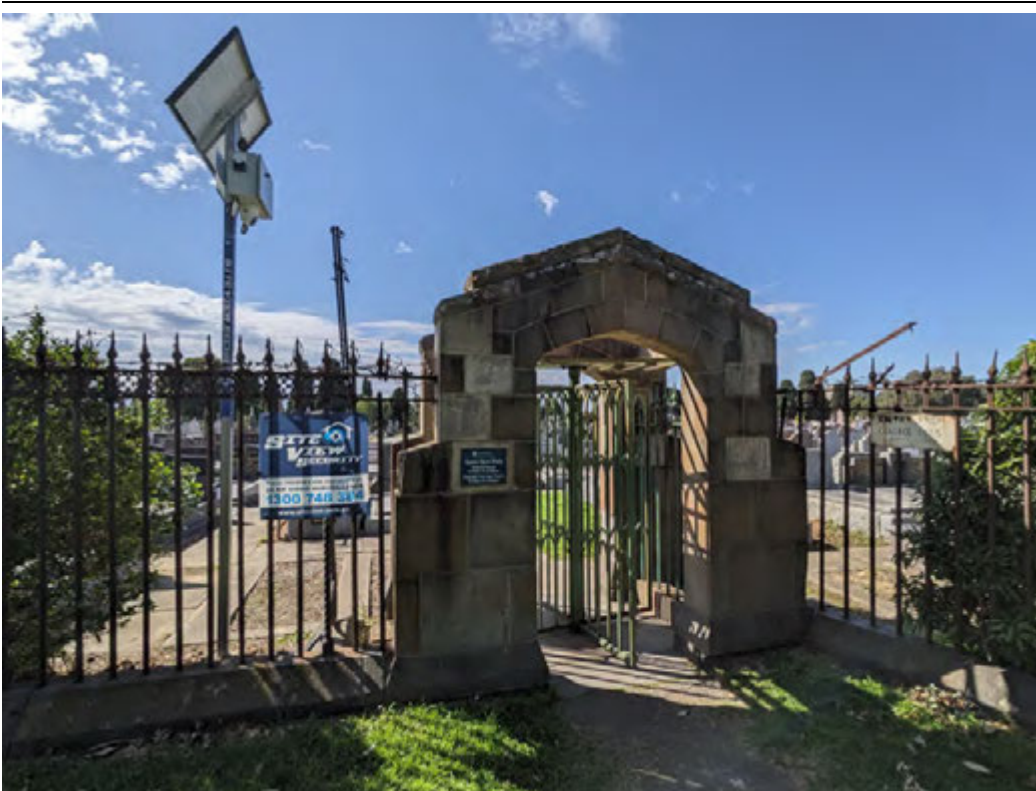
Figure 2 West cemetery gate viewed from the west showing sandstone arched opening and wrought turnstile
