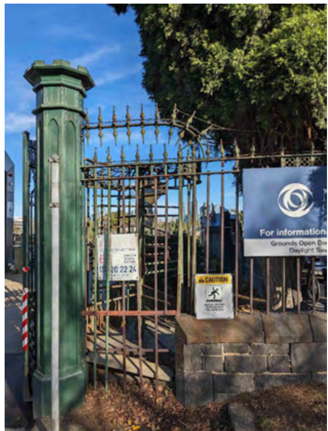
Figure 3 Western turnstile pedestrian gate
