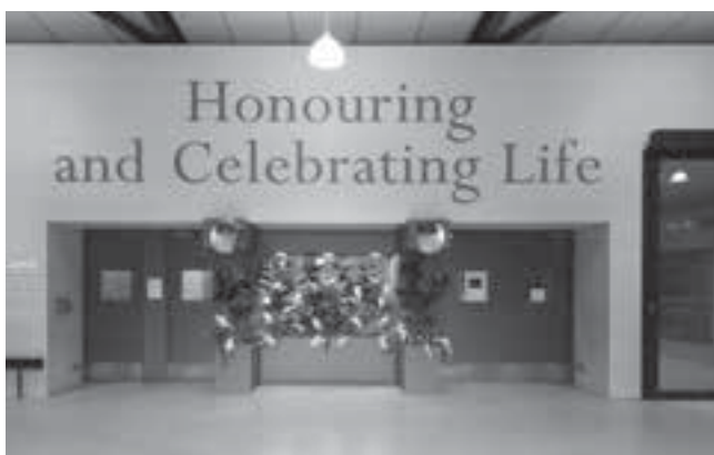
The exterior of the recently refurbished Witness Cremation Viewing Room at Springvale Botanical Cemetery
