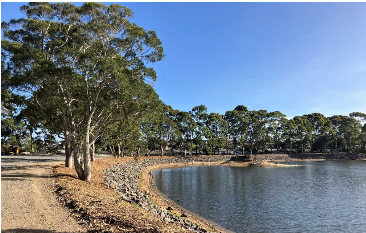
SMCT harvests stormwater for irrigation use at Springvale Botanical Cemetery
